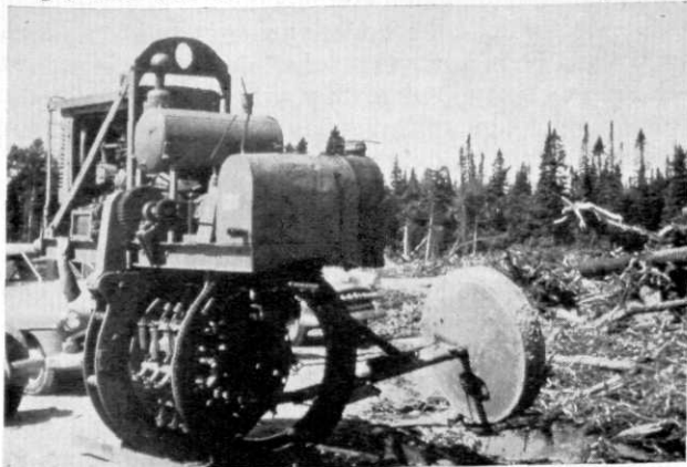
Pipe washing machine designed for the pipes used in the crossing.
