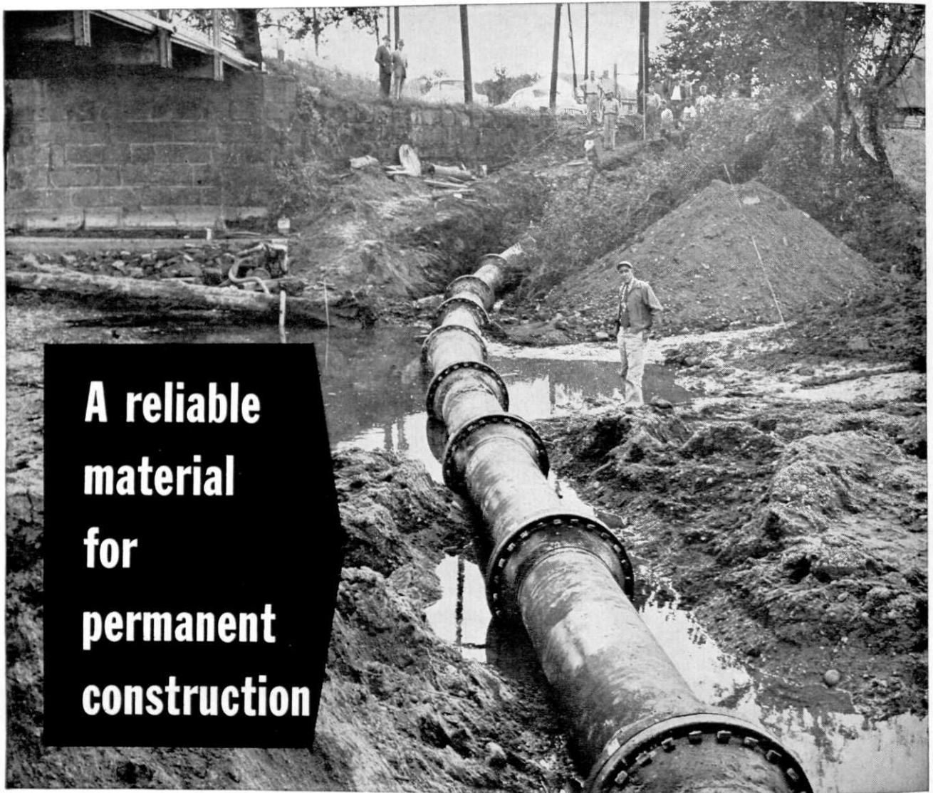
Ball-and-socket joint cast iron pipe for water main crossing river at Newark, Ohio.
