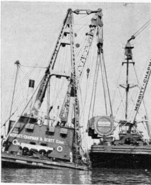
**HALF-MILLION POUND PACKAGE—**Tilted by the tremendous weight of the huge 467,000-pound generator stator for the Boston Edison Company's Mystic lower station, Everett, Mass., is the MONARCH, the heaviest lift commercial derrick on the east coast. It required nearly the maximum lifting ability of the MONARCH to lift the generator stator and place it on the deck of the reinforced-hull derrick CATSKILL.
