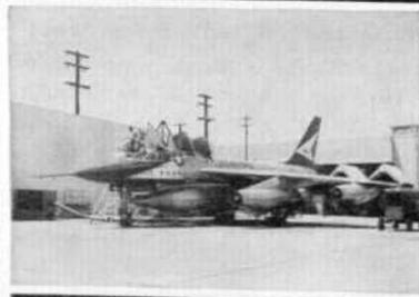
Final checkout of B-58 is performed with special 50-ton refrigeration unit to cool electronic equipment, and an electric-power generator.
