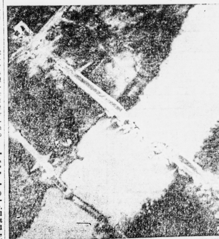
These two bridges across the Volturno river in Italy were wrecked by the Germans in an effort to prevent a crossing by Allied troops. This photo was made from a reconnaissance plane. (AP Wirephoto.)
