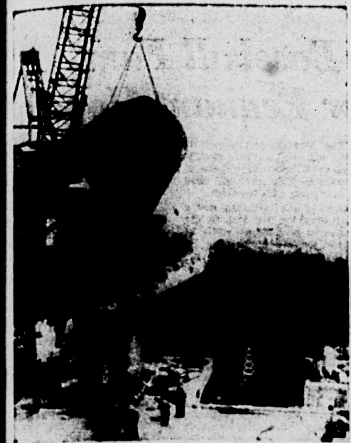
WEIGHING 70 TONS, 56-foot-high bow of nuclear-powered guided missile cruiser U.S.S. Long Beach is hoisted into place for loading to the powerful ship under construction in Quincy, Mass. Navy's first atomic surface ship, 721 feet long, will be christened July 20.
