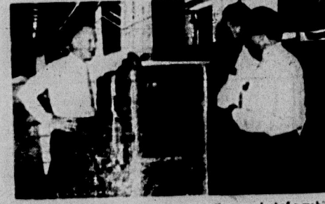
"1:00 p.m. After lunch, I drive out to the new plant of a mobile home manufacturer. My men are completing installation of a new-type cordless switchboard. I discuss features of the new equipment with the firm's Vice President and Plant Manager."
