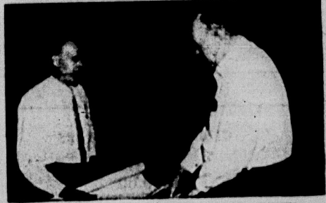
"8:00 a.m. I meet with one of our Foremen at the plant garage to discuss a cable-pneumating job. We're putting all aerial cable in Hutchinson under air pressure to keep out moisture which causes cable failure and costly service interruptions."
