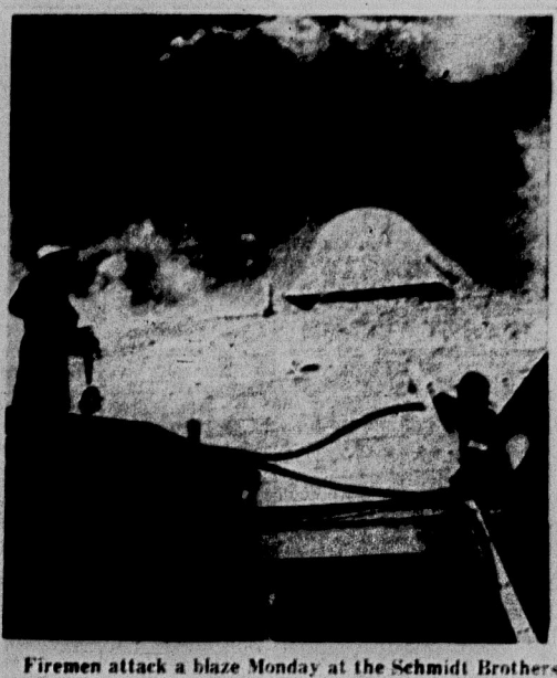
Firemen attack a blaze Monday at the Schmidt Brothers supermarket, which caused damages estimated between $100,000 and $140,000. The smoke and fire attracted nearly 5,000 spectators. State News Photo.
