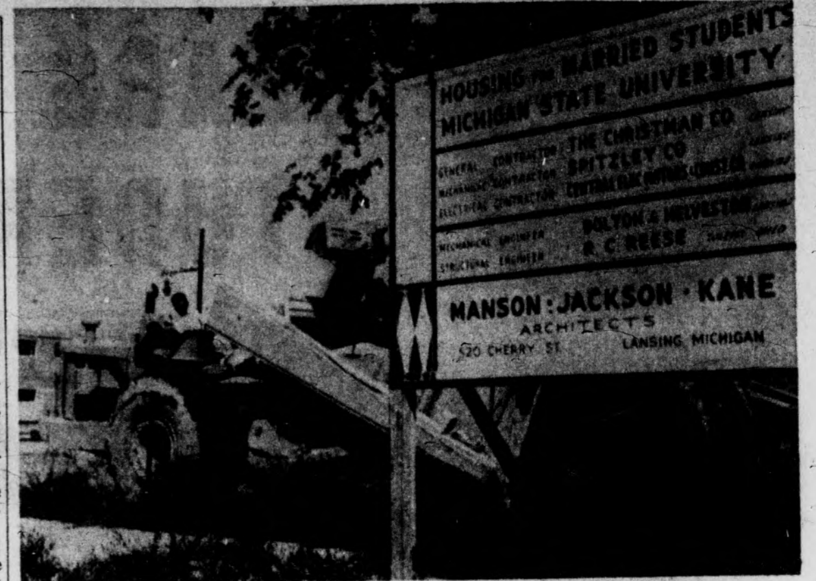
Progress has been slow on the 116 unit addition to the Cherry Lane apartments, part of the university's married housing facilities. Thirty-six apartments, in four buildings, are expected to be ready for occupancy next week. After that, two buildings are scheduled to be completed every two weeks.
