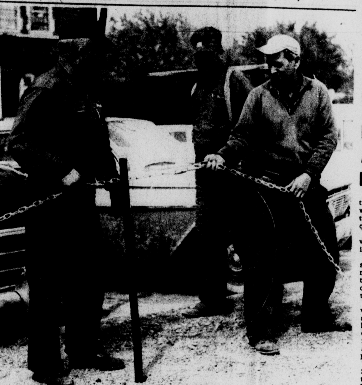
Maintenance crews are beginning the awesome task of preventing students from breathing a path across the campus grass. Here, three men are erecting a chain fence across the street from Barker hall.
