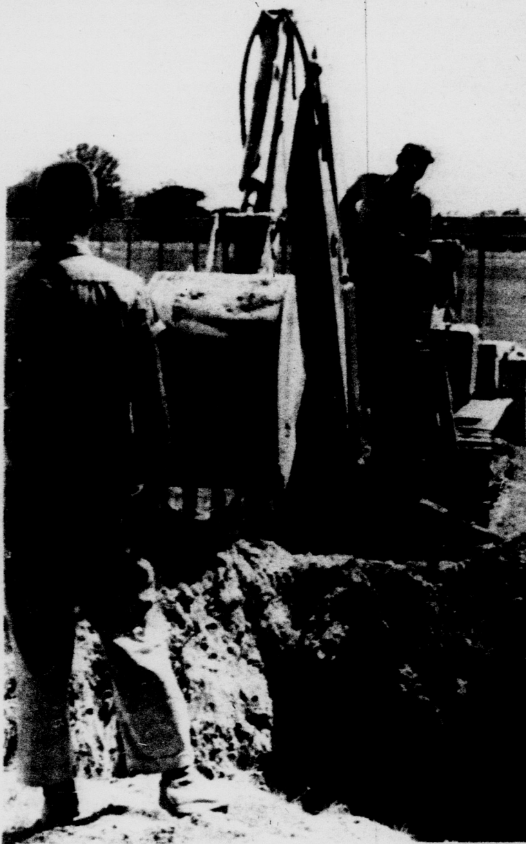
ROAD WORK BEGINS --Motorists using Shaw and Farm lanes will be ducking cranes, tractors and workmen all summer as construction crews begin street widening projects on both thoroughfares and repair steam tunnels along them.
