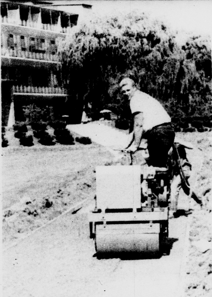
DIRT PATHS ARE OUT- Paving the beaten paths, such as between Farm Lane and Kresge Art Center, is now in progress as campus crews endeavor to keep the campus green. --State News Photo.
