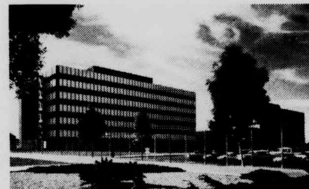
Modern Facilities More than $50 million have been invested in Astronautics' plant and equipment. Complete laboratory, test and computer facilities are established in-plant to enhance the performance of Astronautics' engineering tasks.
