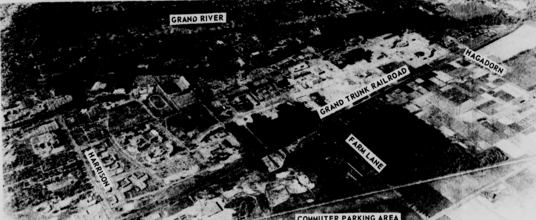
EFFECT OF DRIVING REGS -- With driving to be prohibited on campus in an area marked by Grand River Avenue to the north, Harrison to the west, Hagadorn to the east and the Grand Trunk railroad tracks in the south, and restricted access routes, the new commuter parking lot, bottom right, will have to be constructed over the summer. An express bus service will transport riders to campus.
