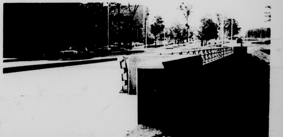
THE ICEMAN COMETH -- But this year when the Red Cedar freezes over, there won't be as many students taking unscheduled swims in the icy waters while taking a short cut. The reason is the new Bogue Street Bridge which officially opened this week. Photo by George Junne
