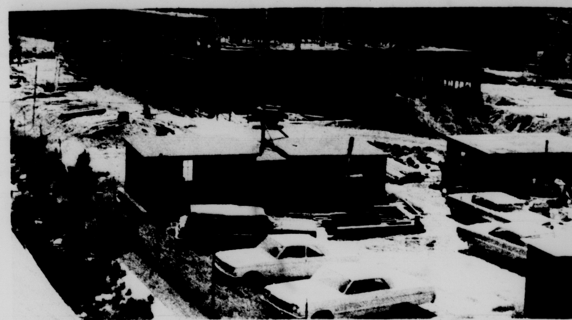
BLOSSOMING near Snyder-Phillips Halls is the northeast section's share of the latest campus construction program, the new $350,000 Psychology Building, to be completed in December.
