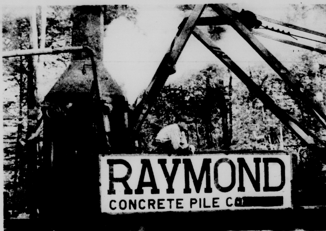
RELIC—This steam pile driver, replaced more often today by diesel power, is being used on construction work for Owen Graduate Center's addition. Photo by Ken Roberts
