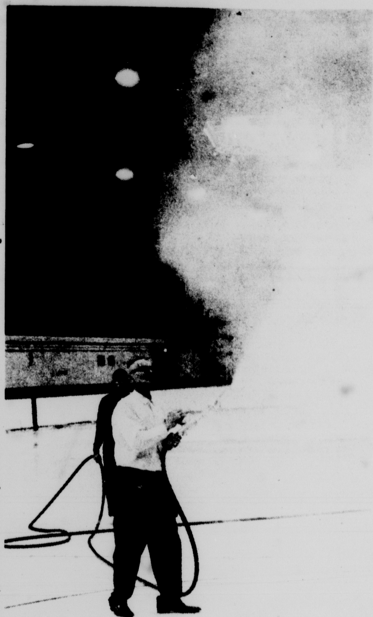
WET PAINT FOR WET ICE-- The freshly-painted lines on the first protective layer of ice are being protected by John Duncan, as he gets the rink ready for hockey action. The water will prevent the paint from being smeared when the ice machine lays the successive protective layers. Photo by Jim Hile
