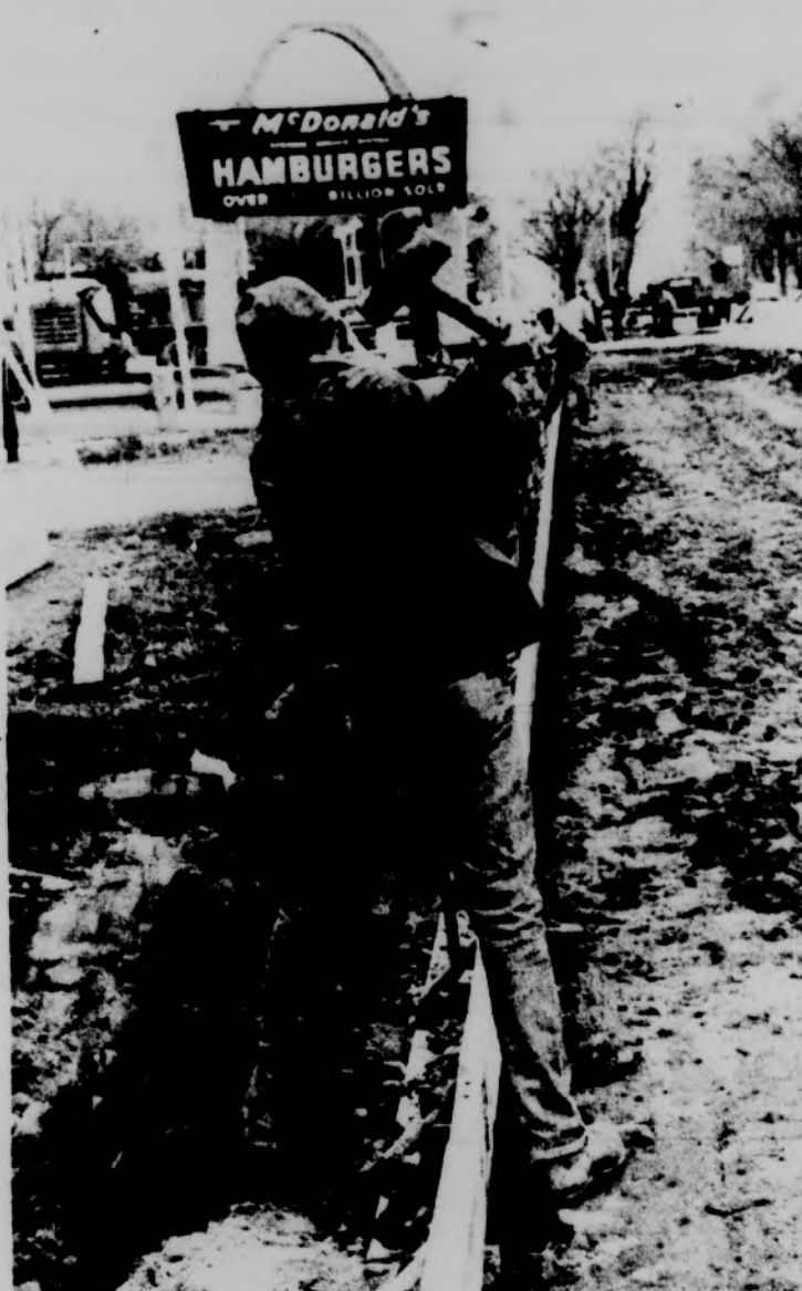
HOW GRAND—Construction continues just off the Michigan State campus on Grand River Ave. to widen the road for more lanes to carry the large amount of traffic that centers around MSU. The widening process will also make way for sewer pipes for the East Lansing area.
