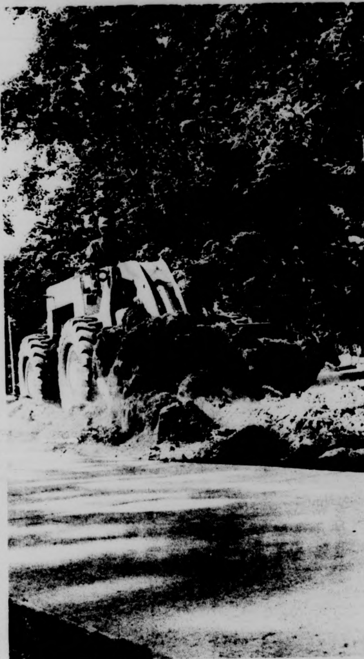
SIDEWALK CONSTRUCTION --The new sidewalks and curbs around West Circle Drive are finished. The next step is replacing the dirt around the edges of the sidewalks. This workman is making a back-breaking job easy.
