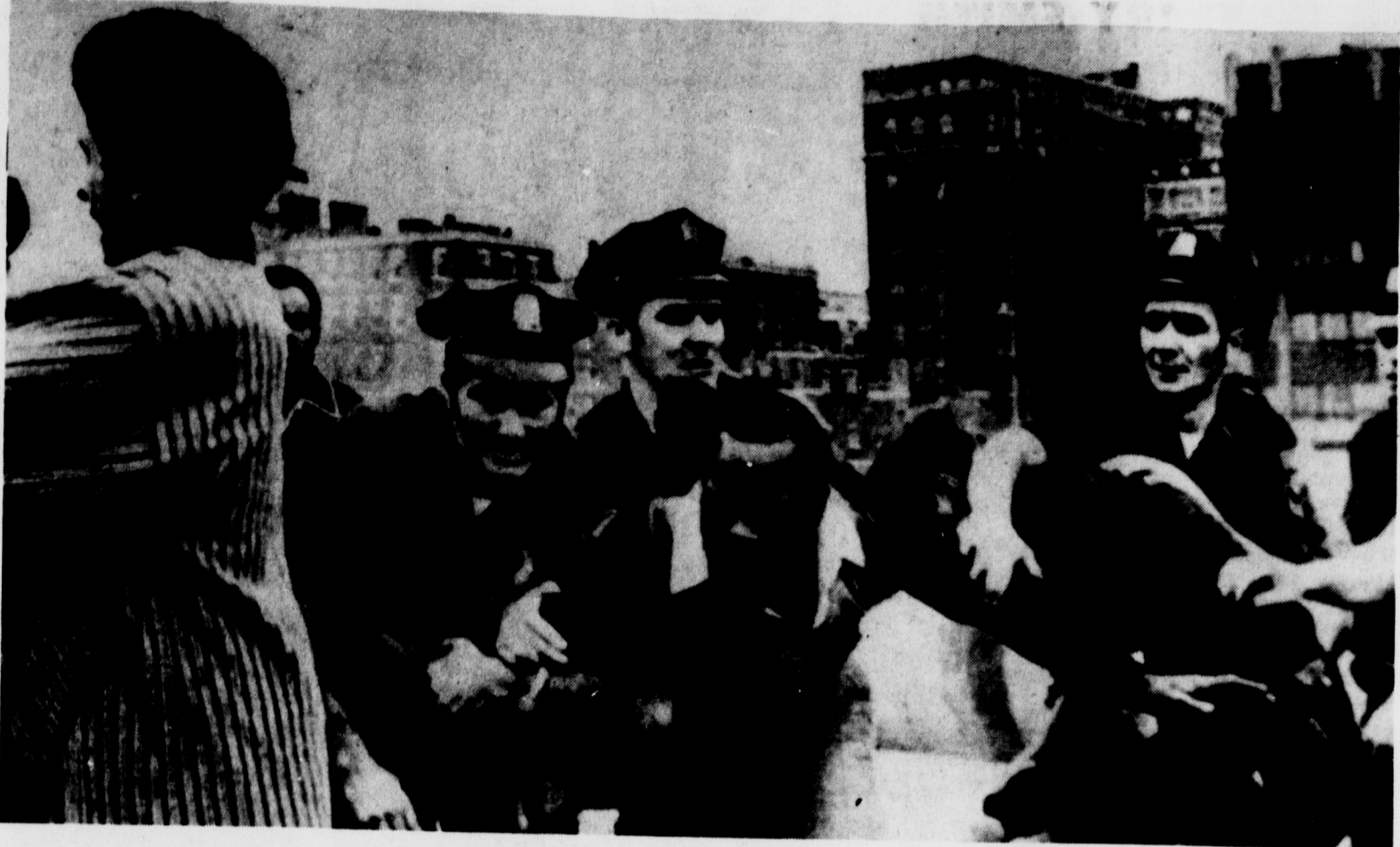
Police haul away a protestor from a construction site at Boston City Hospital Thursday as a group tries to stop a truck from entering the area. Sixteen men and a woman
