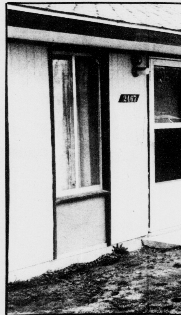
These motel - like structures housed impoverished people at the reservation. Ten years ago through federal assistance. Because
