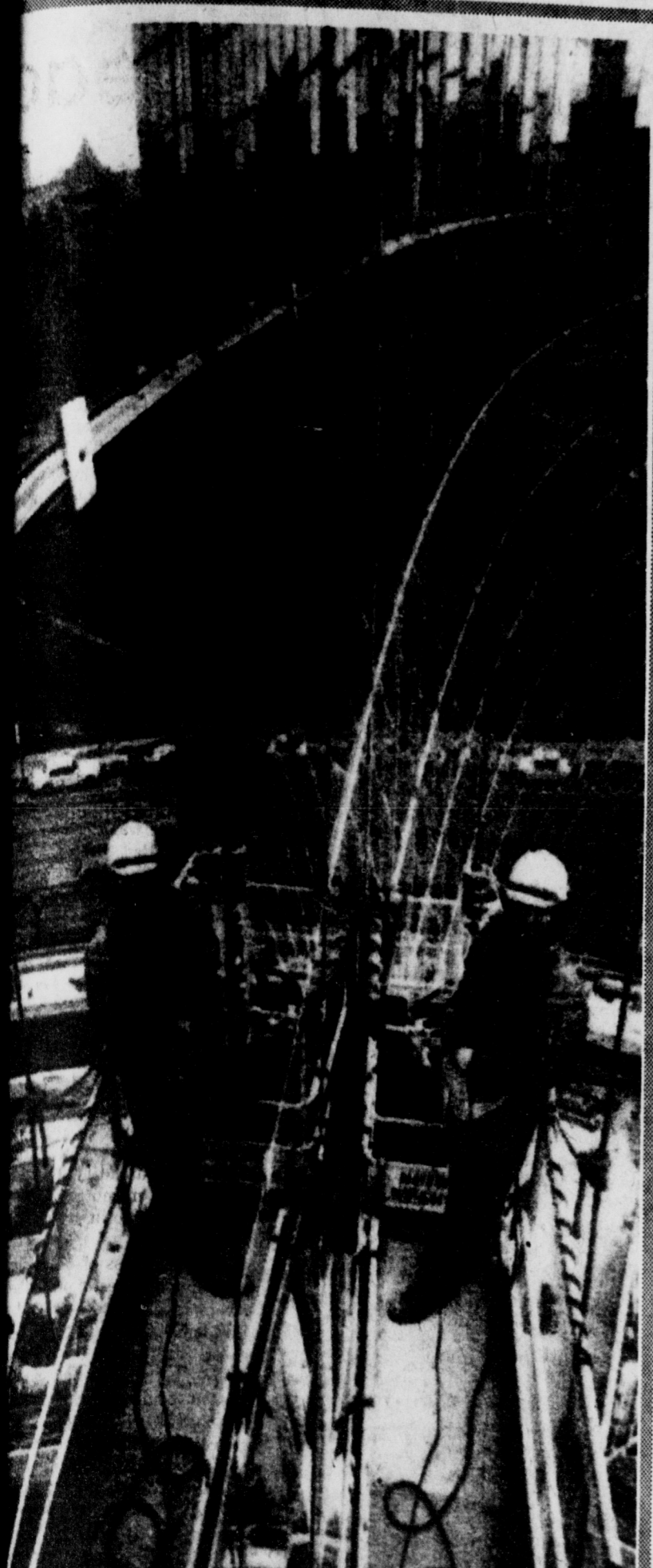
AP wirephoto Construction workers put a mirrorlike siding on the exterior of $44 million Ontario Hydro headquarters in Toronto. The Ontario Legislature is reflected in the glass at left. The building expected to be finished by the end of May.
