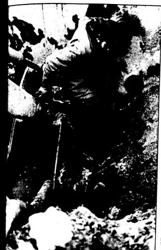
U Physical Plant worker Robert Pitchford labors in the wet, partially en ground near Bessey Hall to repair a water main which burst
