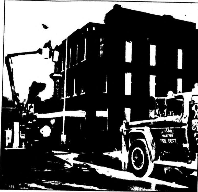
Firefighters battled an early morning fire that destroyed a hotel in Jellico, Tenn., killing at least seven persons and injuring 15. Many of the victims were elderly, permanent residents of the hotel which was built near the turn of the century.
