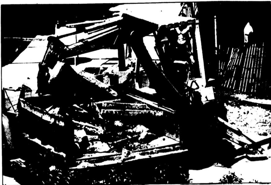
The Wells Hall bridge was the sight of some minor repair work this past week. Workers are replacing sections of the sidewalk that were damaged by snowplows this past winter. Freezing temperatures also expanded the ground moisture, thus raising the pavement in some areas.
