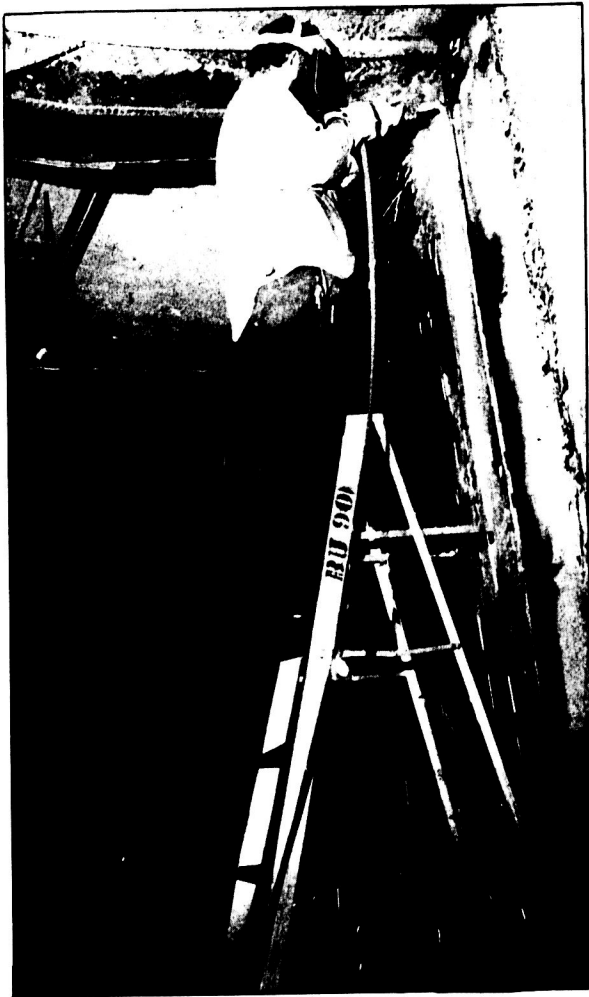
State News/Susan Turo Andy Chrissey, from the physical plant maintenance service, helps upgrade the heating system for the MSU Museum. In compliance with the energy conservation program, the new system operates on less electrical energy.
