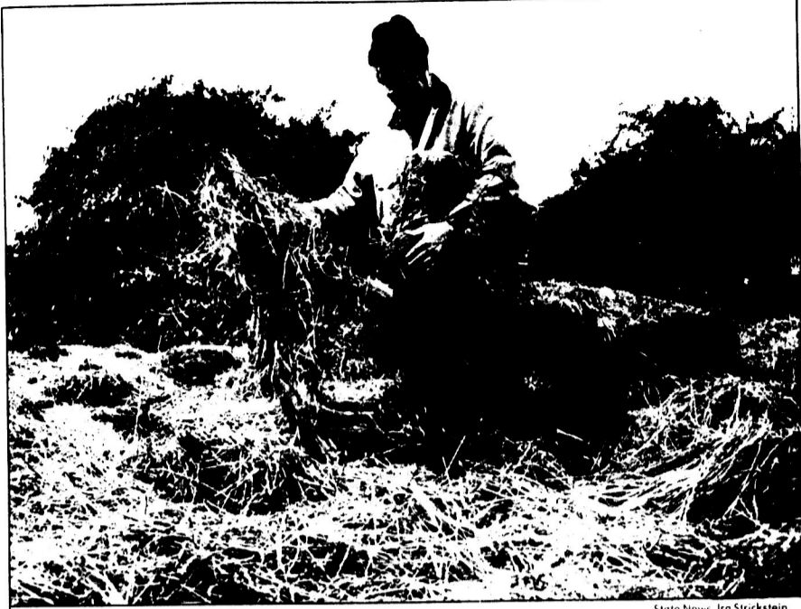
"Smokey" Stover, from MSU Grounds Maintenance, used 60 bails of straw to put the Horticulture fountain to bed for winter. The straw is used to absorb moisture and help prevent cracks in the concrete.
