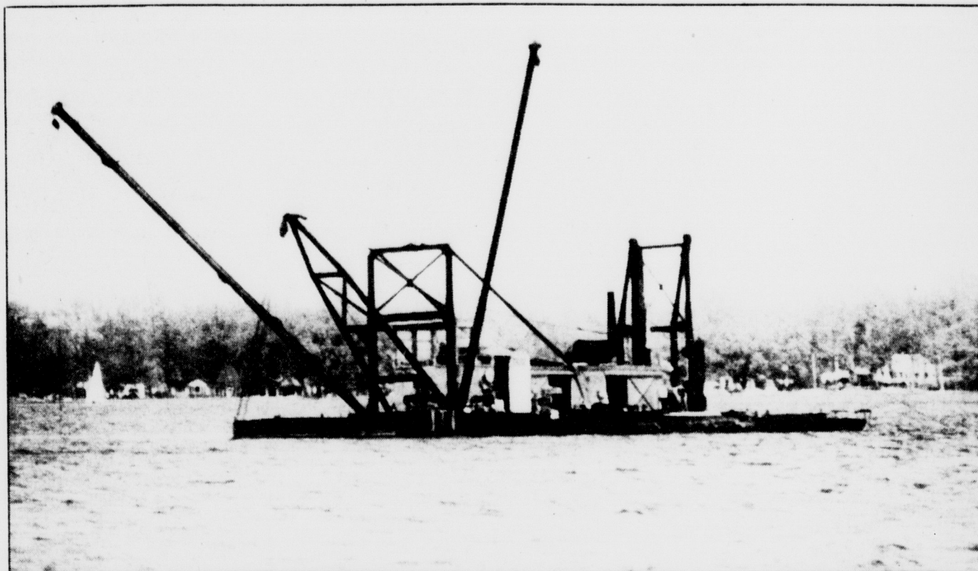
A hydraulic dredge began removing sediments from the bottom of Lake Lansing Thursday afternoon to begin restoring the lake and improving its recreational facilities. State News: Susan M. Pokrefsky
