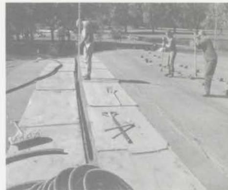
Laser level confirms trench grade; sod tamping begins.
