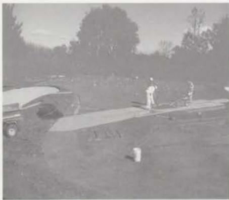
Trencher making 3" x 15" excavation from plywood
