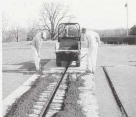
Four-wheeled carts remove excavated material.
