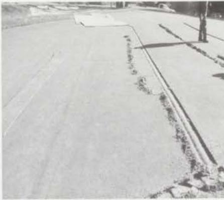
*Trench line ready for sod. A trench compaction compensator tool leaves high spot along trench to allow for slight settling.*
