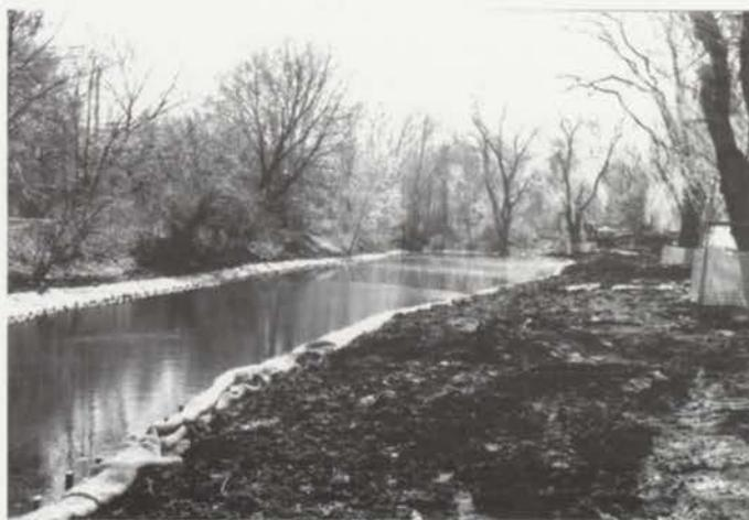
**Middle:** Basin Construction in Progress, Showing Bank Stabilization
